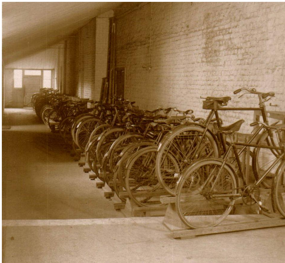
The Bicycle Gallery between the swimming pool and the bath house.
